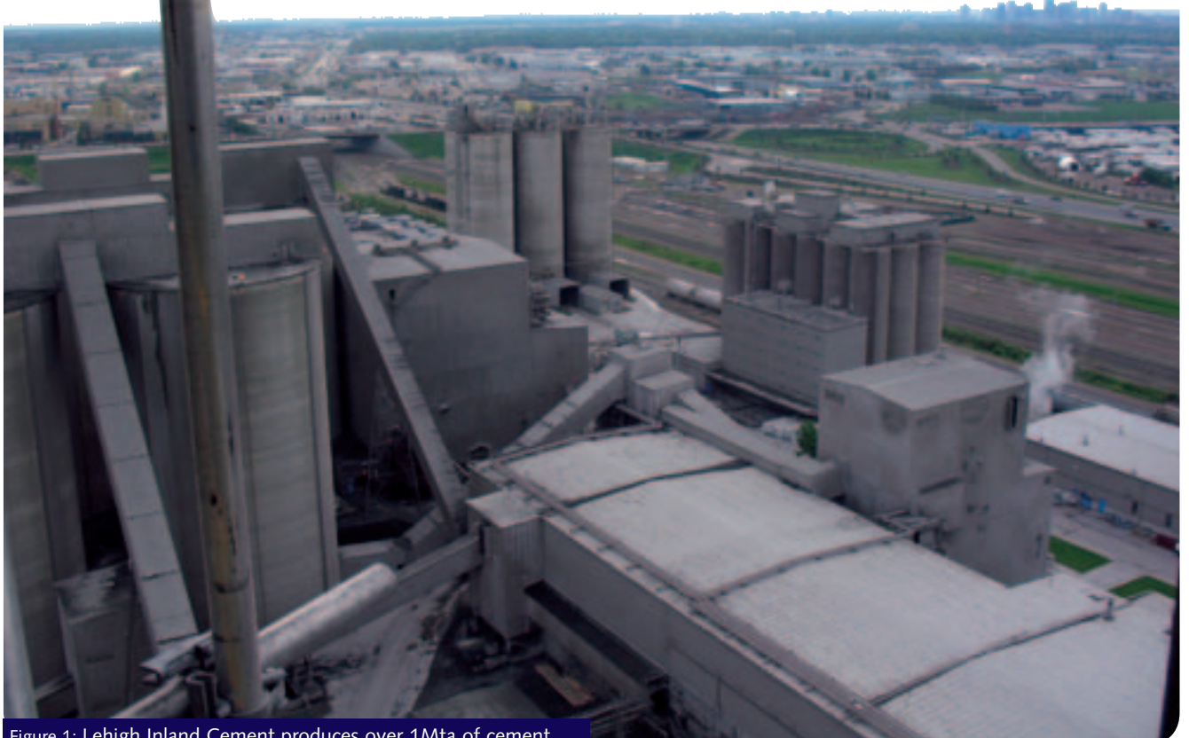
Figure 1: Lehigh Inland Cement produces over 1Mta of cement
